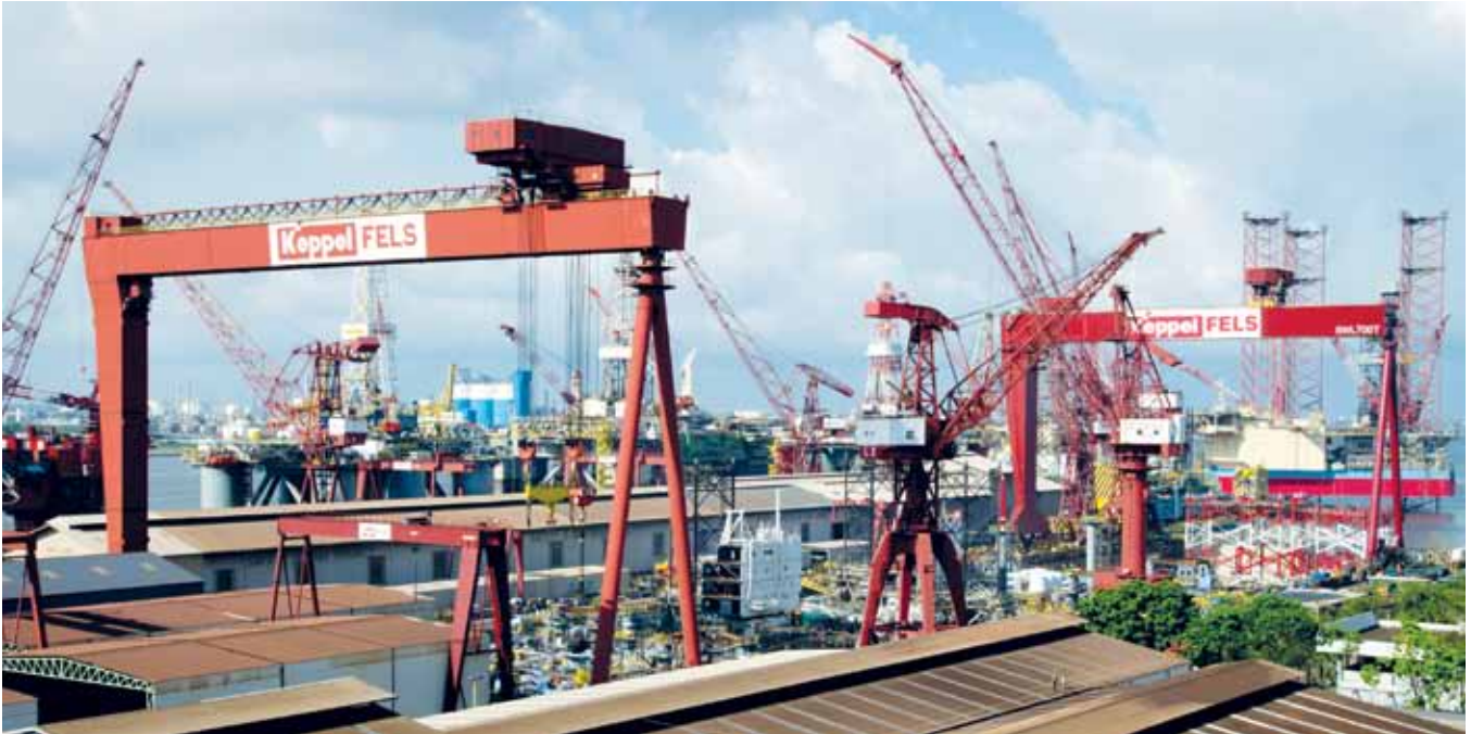
Keppel FELS significantly increases its lifting capabilities with the new 700-tonne gantry crane (right) which adds to its existing 500-tonne crane (left)
